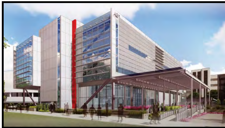
Picture Above: Advanced Engineering Building (AEB)
