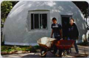
Brothers Derrick Cheng and Janine Watson at work renovating the domes
