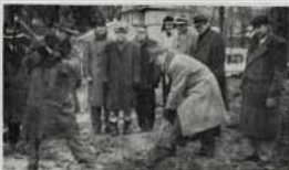
Ground Breaking Ceremony
