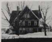
Beta House Repainted
