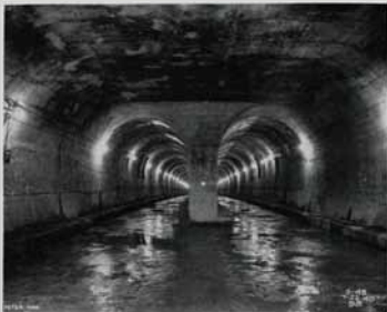
Completed twin tube section at a junction with a crossover section
