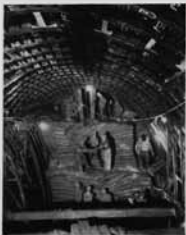
Bench mining operation for the twin tube section
