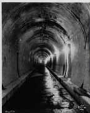
A completed portion of arch section train tube
