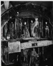
Rear view of the shield in operation
