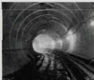
A curve on a section of subway built with shield
