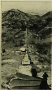
ARC WELDING, GUADALUPE POWER PLANT, PENIXOCA
